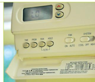
Setting your thermostat to the "On Position" allows your fan to circulate air continuously when not in a heating or cooling mode.
