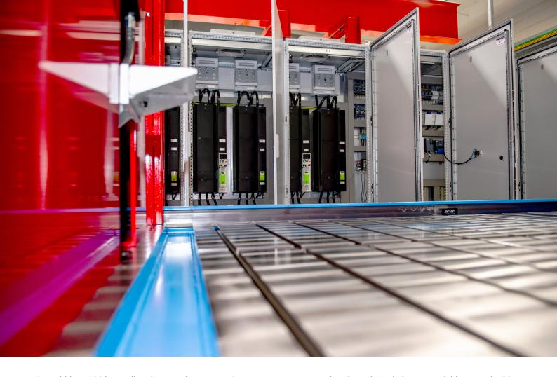
The Unidrive M700 is equally at home acting as an Active Front End (sometimes known as 'regen' or 'grid tie') with voltage boost facility, it has a DC source which can be buck or boost, plus it can act as bi-polar and bi-directional or a motoring/ absorbing drive. Current and speed loops are all synchronised with current loop execution in as little as 62.5us, and the switching frequency on the 320 amp modules is up to 16kHz.
