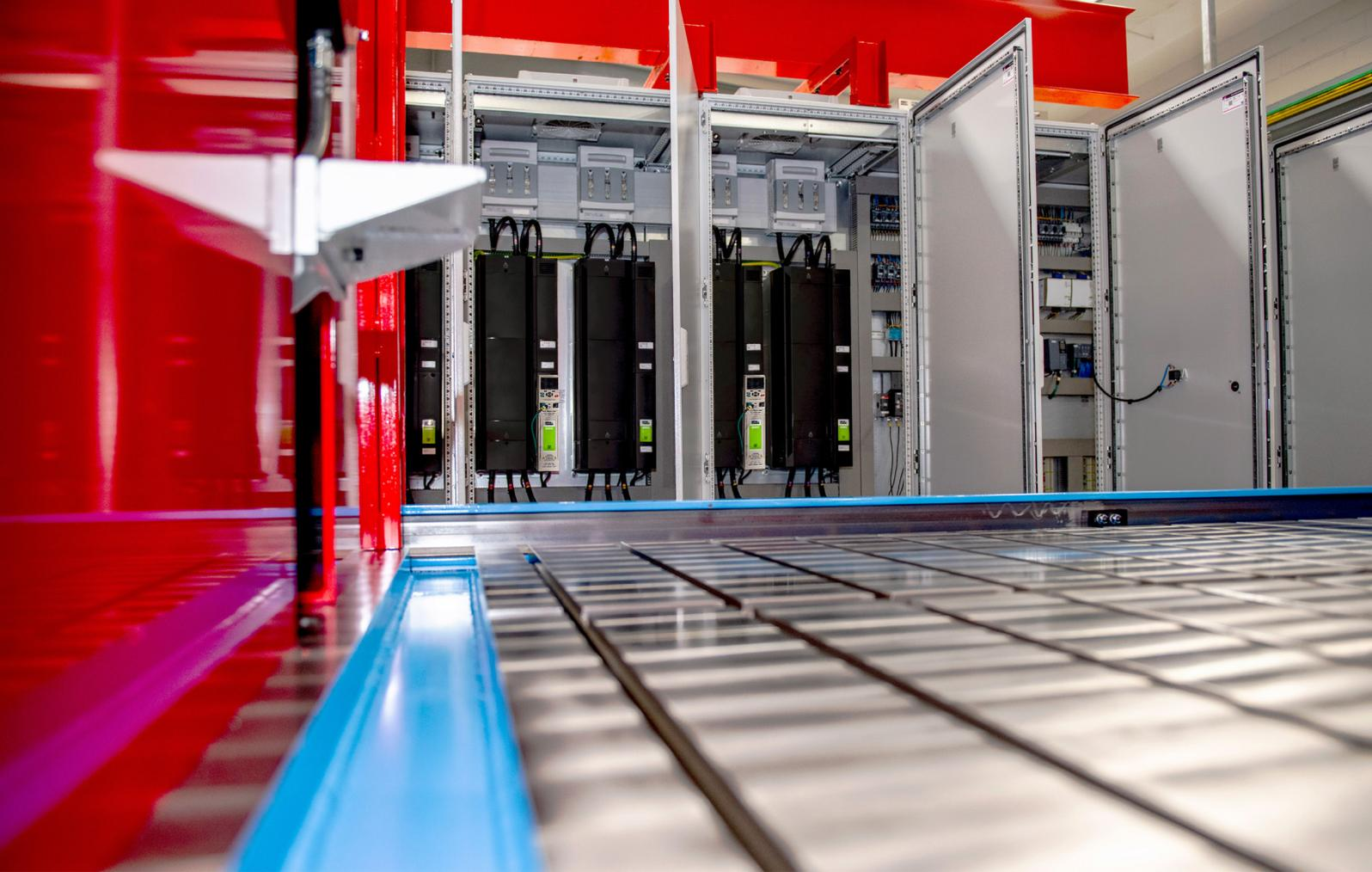
The Unidrive M700 is equally at home acting as an Active Front End (sometimes known as 'regen' or 'grid tie') with voltage boost facility, it has a DC source which can be buck or boost, plus it can act as bi-polar and bi-directional or a motoring/absorbing drive. Current and speed loops are all synchronised with current loop execution in as little as 62.5us, and the switching frequency on the 320 amp modules is up to 16kHz.
