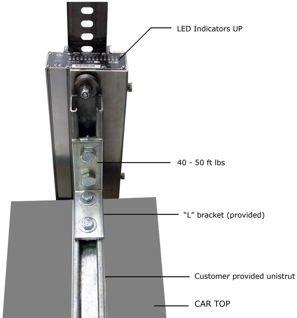
**Sensor Alignment** After the tape has been installed, check the sensor alignment. The sensor should not ride hard on either side of the Unistrut bracket during any part of travel through the hoistway. In high-rise buildings, if rail alignment varies substantially, it may cause the encoder guides to wear prematurely. If such misalignment is noted, the installation should be inspected more regularly.
