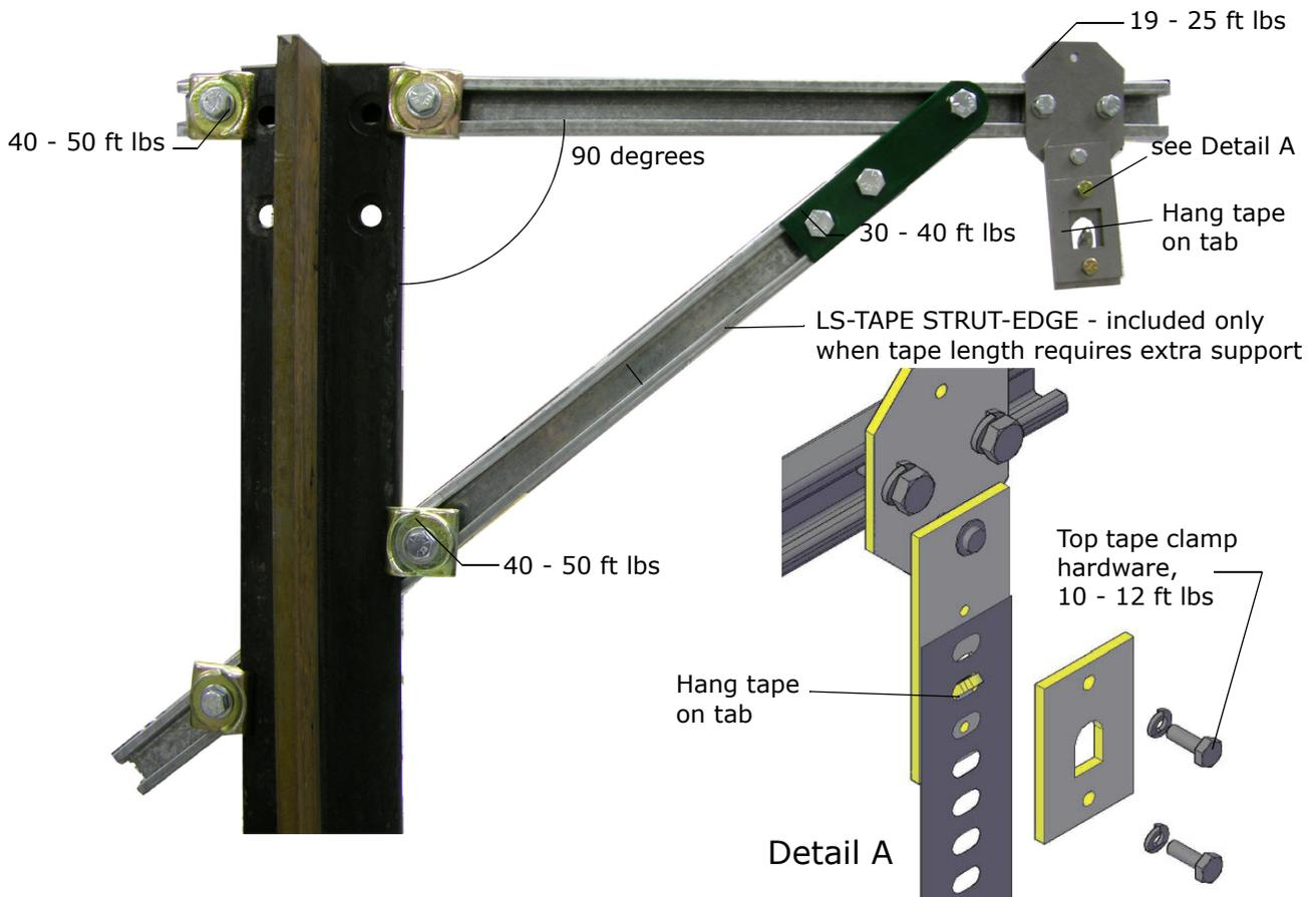
3. Adjust extended strut length as required (tape suspended as close to the guide rail as adequate clearances will allow to reduce loading on end of Unistrut channel). Secure rail mounting hardware (40 - 50 ft lbs.). (The tape hanger slides in the strut for fine adjustment later.)
