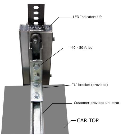
**Sensor Alignment** After the tape has been installed, check the sensor alignment. The sensor should not ride hard on either side of the uni-strut bracket during any part of travel through the hoistway. In high-rise buildings, if rail alignment varies substantially, it may cause the encoder guides to wear prematurely. If such misalignment is noted, the installation should be inspected more regularly.
