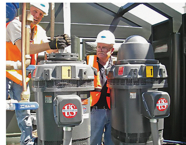
Workers install new vertical motors in Denver, CO.
