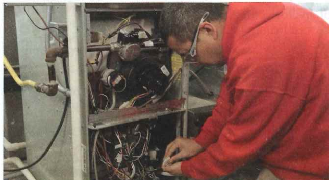
A student at work at Ranken, when the electrical manufacturer Nidec Corp. has invested in a new training facility. —Nidec Motor Corp. photo
