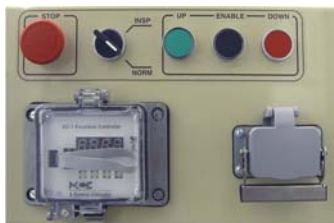
Main cabinet (top view) controls, standard programmer, and inspection control plug
